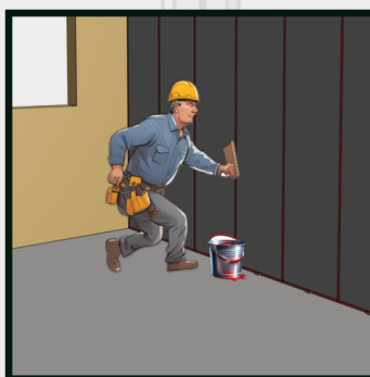
Fill the gap with bonding agent and remove any excess
