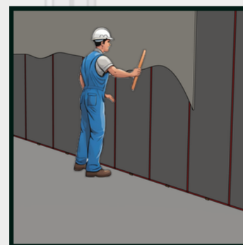
Apply skim coat to the exterior as finishing
